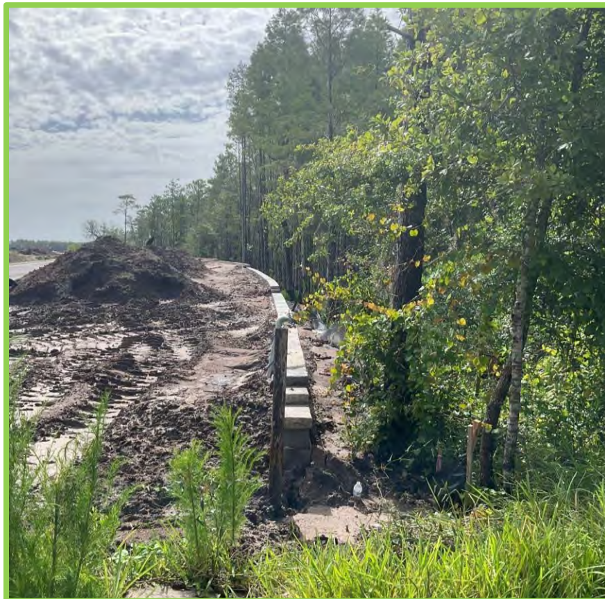
Figure 24. Construction and downed silt fence at N 28.281014, W 82.456108
